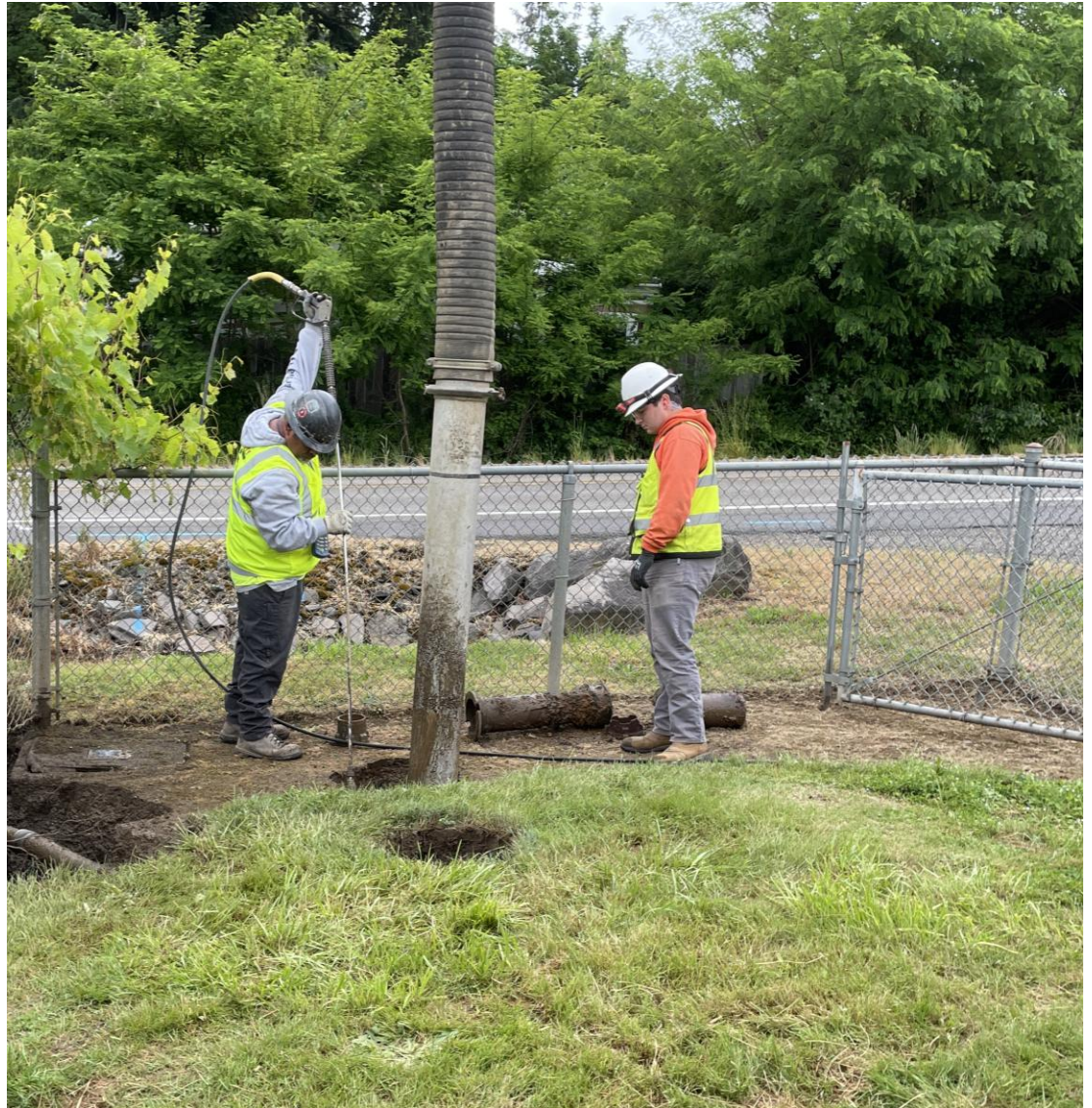
REDLAND PUMP STATION UNDERGROUND EXPLORATION
